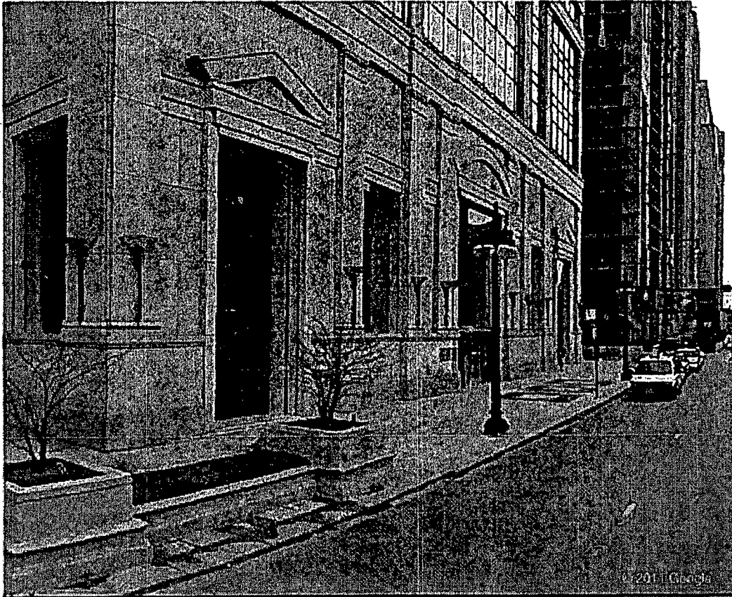
View of United Building
