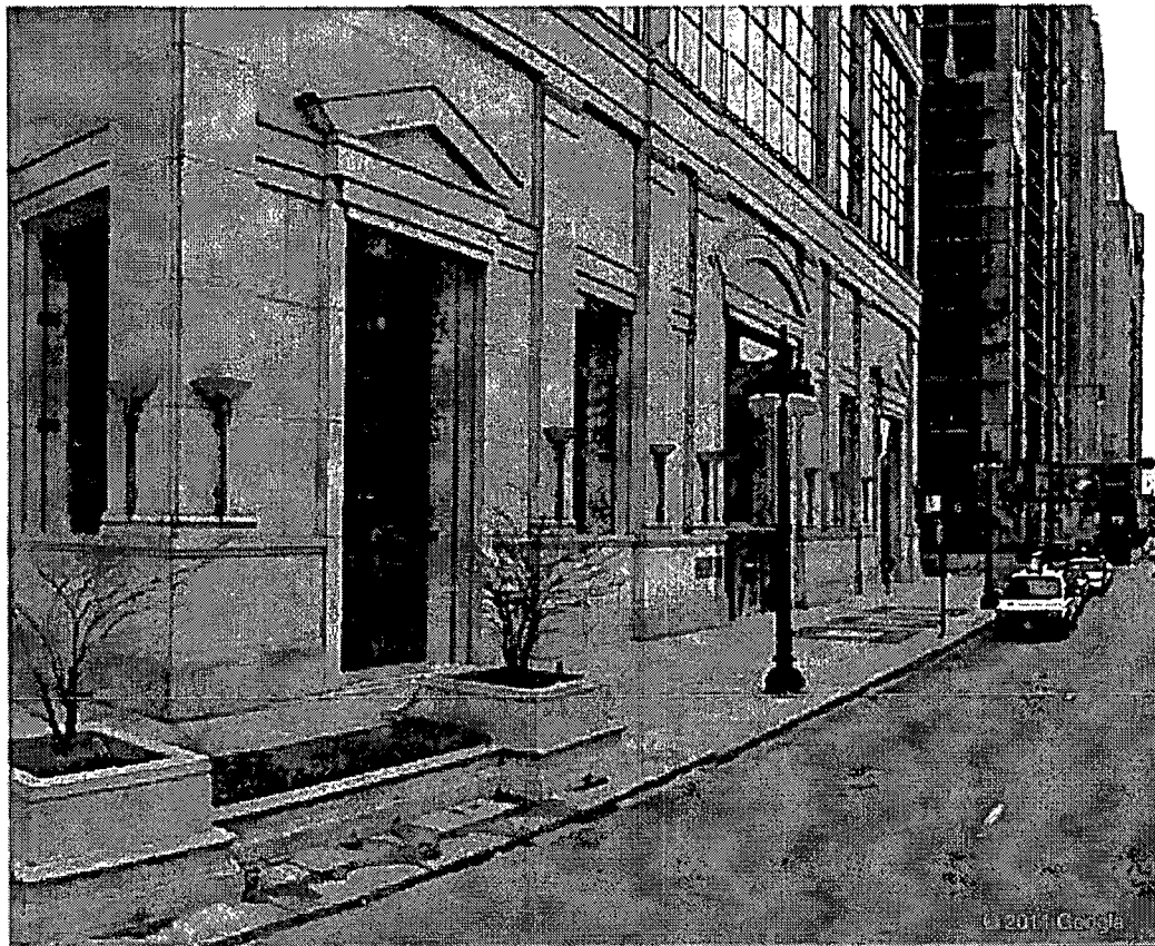
View of United Building
