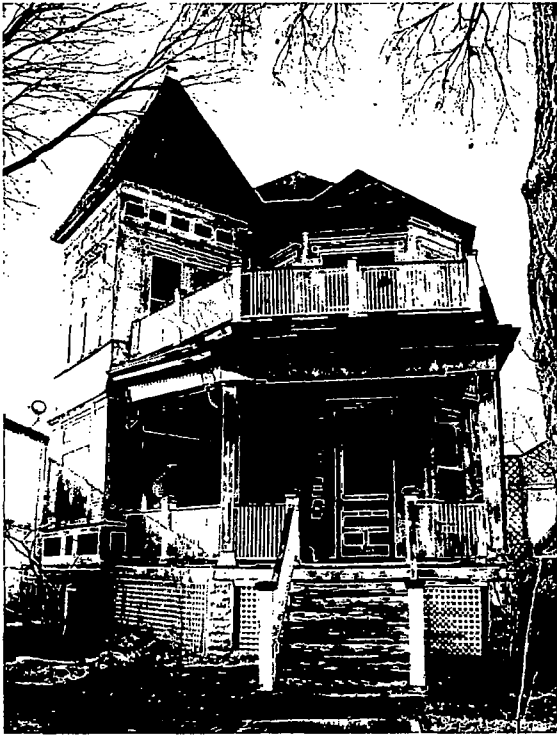
The front elevation of the house features a large corner tower and a raised porch leading to the paneled entrance door set in a projecting bay. The balloon-frame structure is sheathed in narrow clapboard and shingles. Large double hung windows are glazed with clear glass and accented with art glass transoms.
