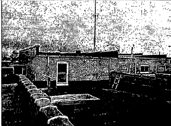
Fig. 21 – Dividing wall between lots 6, 7&8 and the rest of the building on roof, looking toward S. South Chicago Ave.
