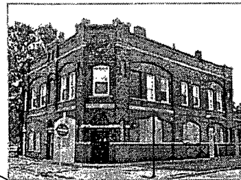
(Former) Schlitz Brewery-Tied House 11400 S Front Ave. Date: 1906 Architect: Frommann & Jepsen (attributed)
