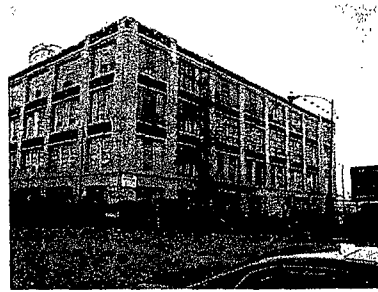
3 PHOTOGRAPH LOOKING AT WEST ELEVATION SCALE: NTS
