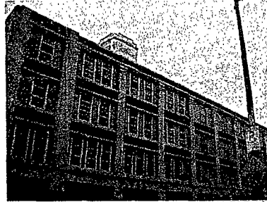
3 PHOTOGRAPH LOOKING AT NORTH ELEVATION SCALE: NTS
