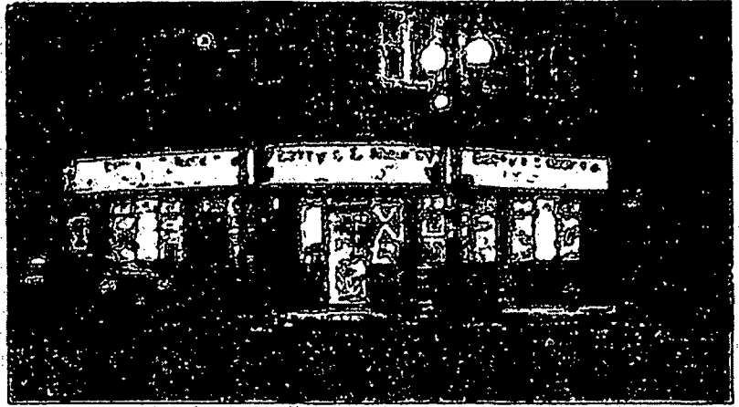
1 Standard Awning constructed of galvanized steel frame 1" square tube Translucent Awning Vinyl sewn and wrapped on awning frame
