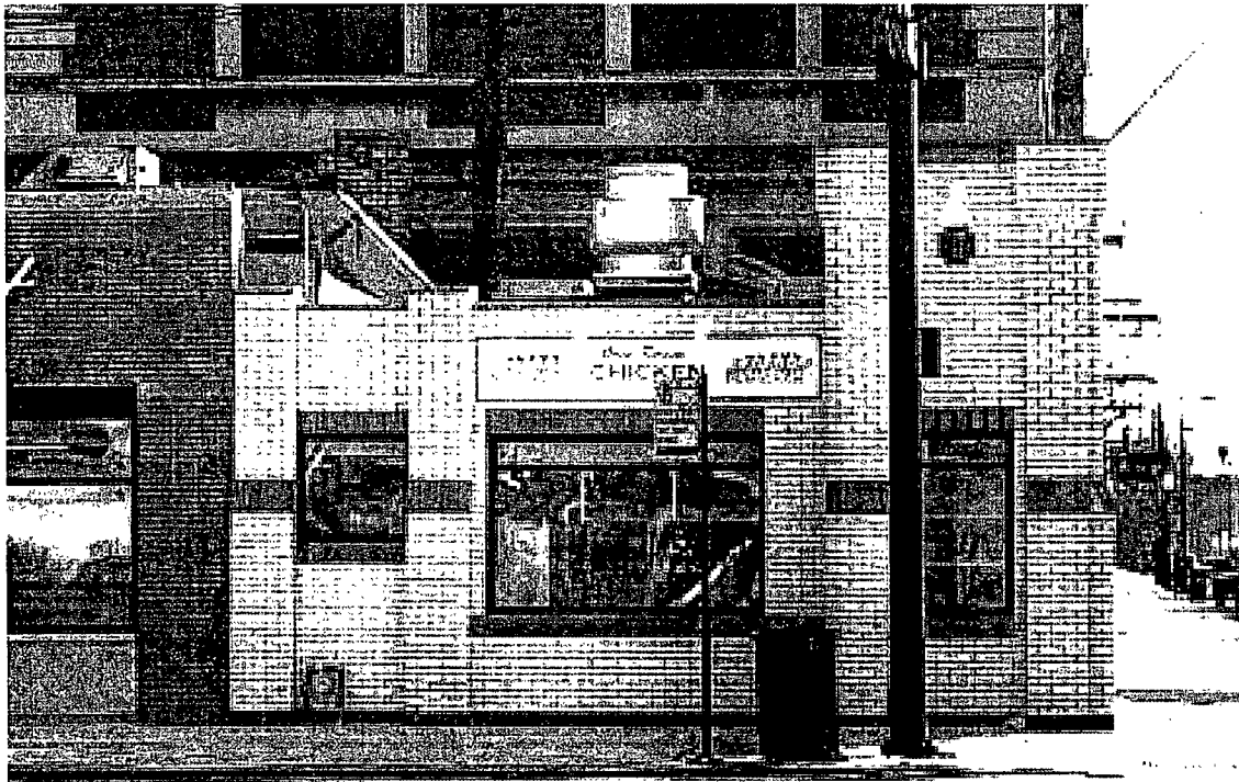
White Castle #16 is a small commercial building built of white-glazed brick with green and beige brick trim. Its corner location, visually-prominent corner tower, and crisp form and detailing give the building a visual scale that belies its diminutive size. The building's design was a standard one used by White Castle in the late 1920s and early 30s.
