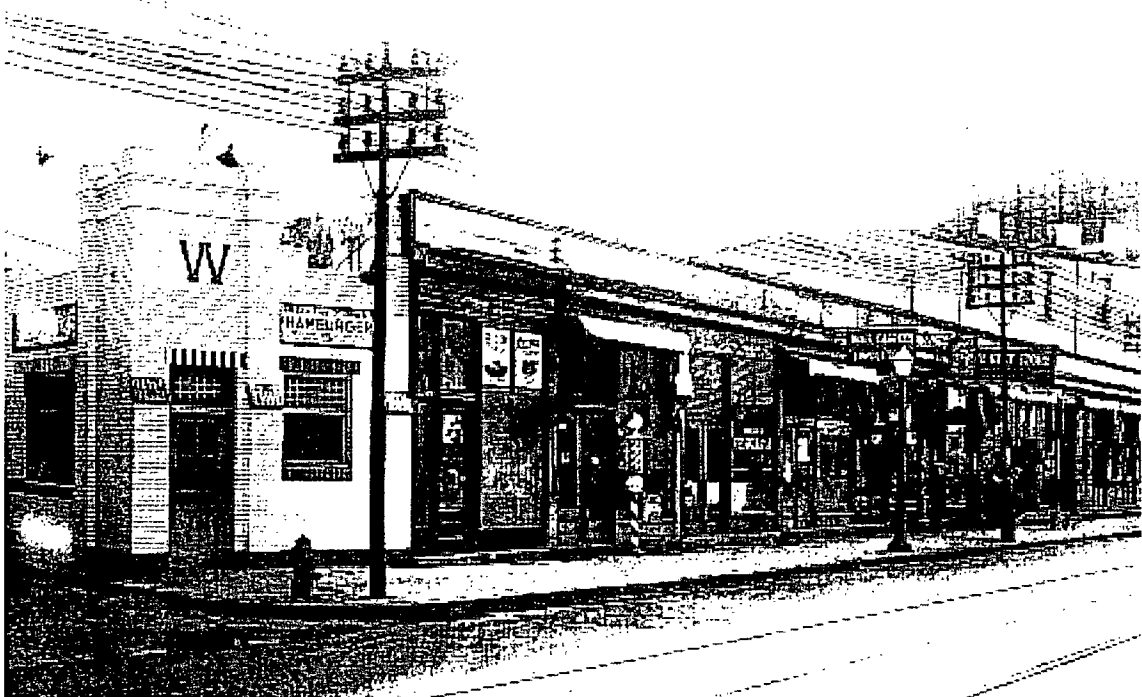
White Castle's buildings are early and significant examples of programmatic architecture, meant to serve as visual "billboards" for the company and to stand out from more traditional streetscapes. Top: White Castle # 5 in Columbus, Ohio, was located in a non-descript industrial area adjacent to downtown. Bottom: White Castle # 9 was a striking visual anchor for this stretch of one-story commercial buildings in a working-class neighborhood of Cincinnati, Ohio.
