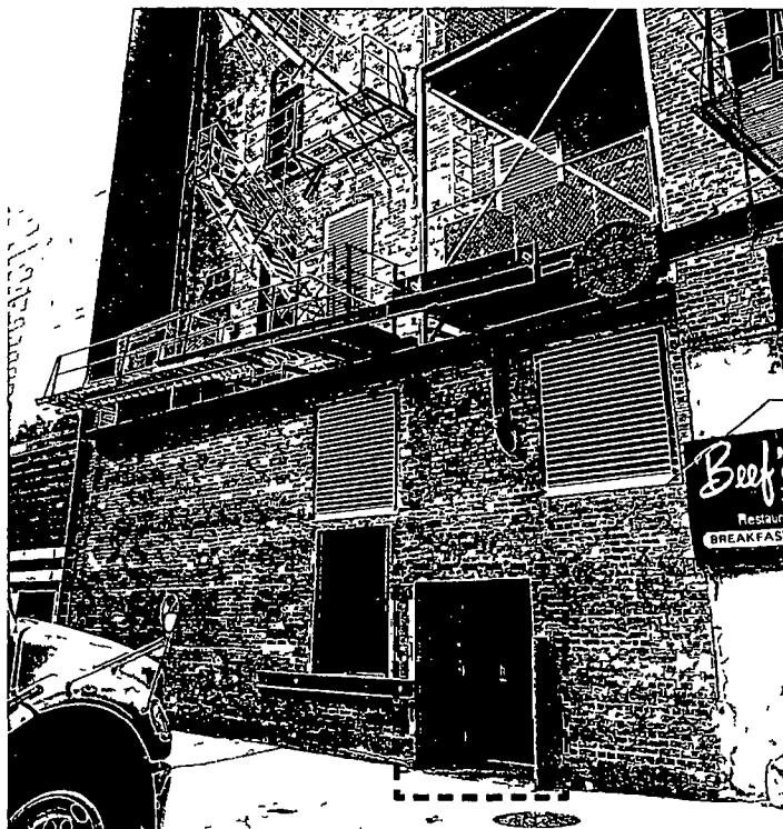
PHOTO OF FACADE - EXISTING SCALE NTS
