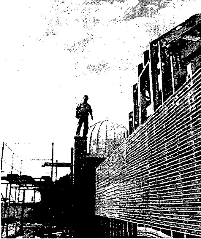
Ron Baltierra, president of Baltierra dr/ Balti, the contractor that built the arch stands atop one of the towers. The span of the arch shows a light-gauge steel structural frame and metal lath prior to application of finishes.
