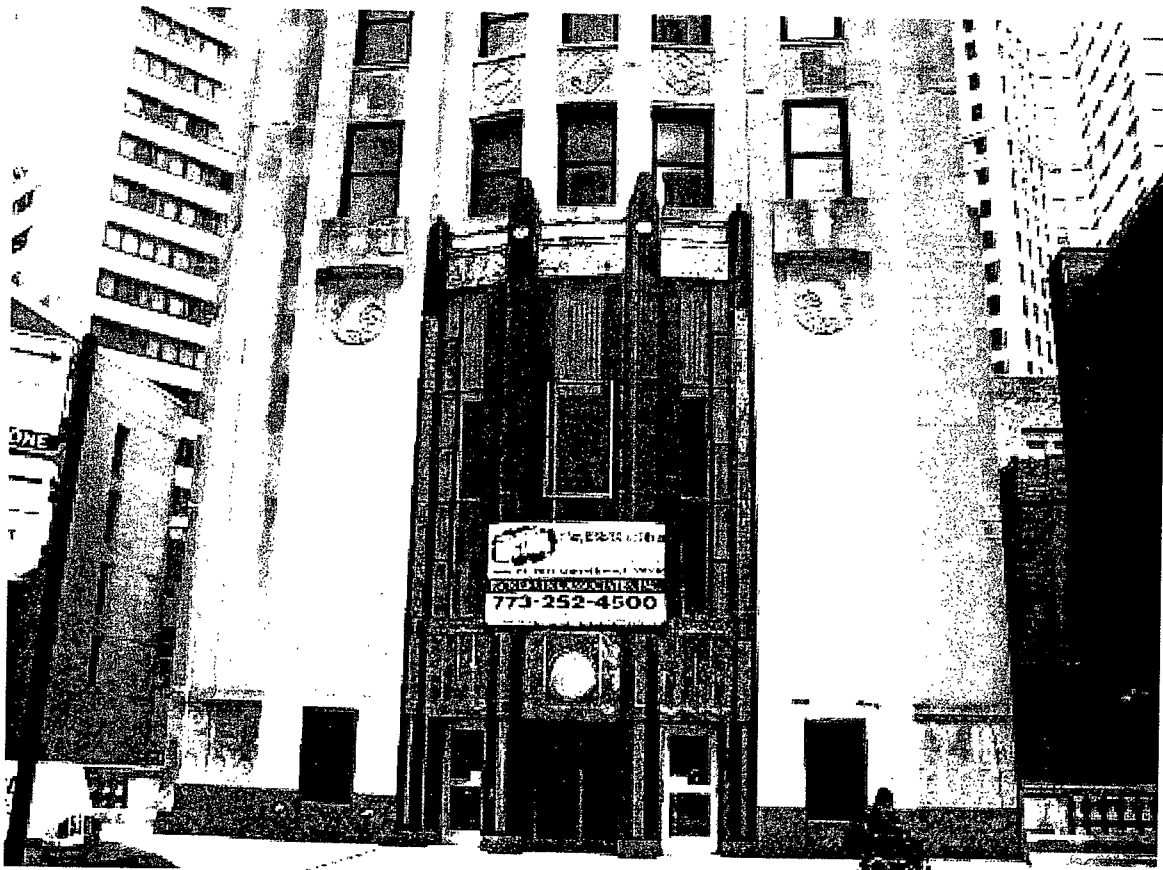
Top: The building's verticality is emphasized by a wide, visually-dominant central bay above the main entrance that bows gently outward and rises to the building's parapet. Bottom: A highly-decorative and dramatic cast-iron surround frames the building's monumental entrance.
