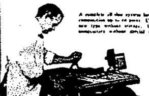
A complete set of this system for direct composition up to 48 lines. Casts most new type without storage. Used by compositors without special training.
