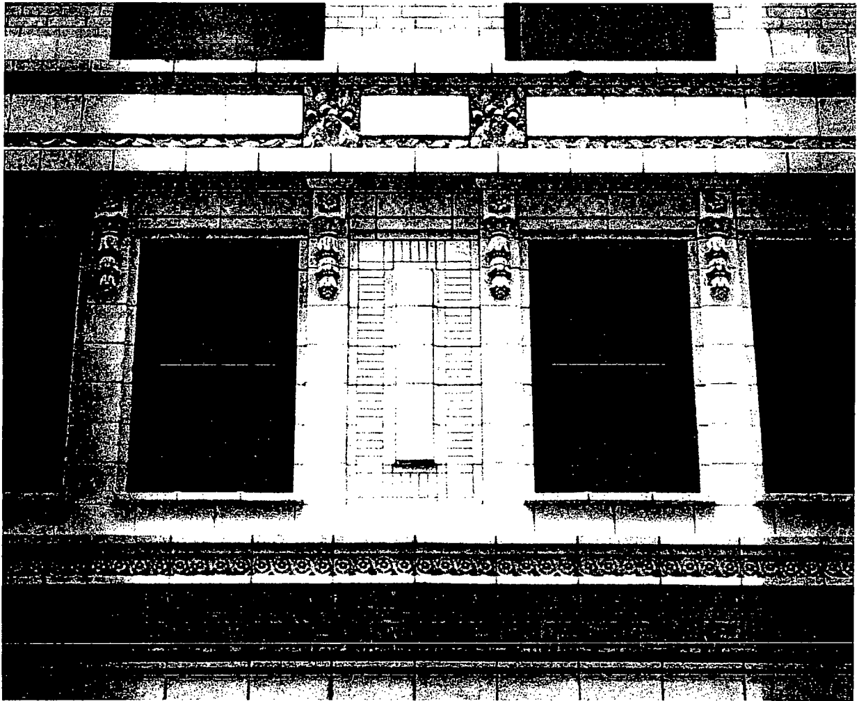
Additional views of the Steger Building's Classical-style terra-cotta ornament.
