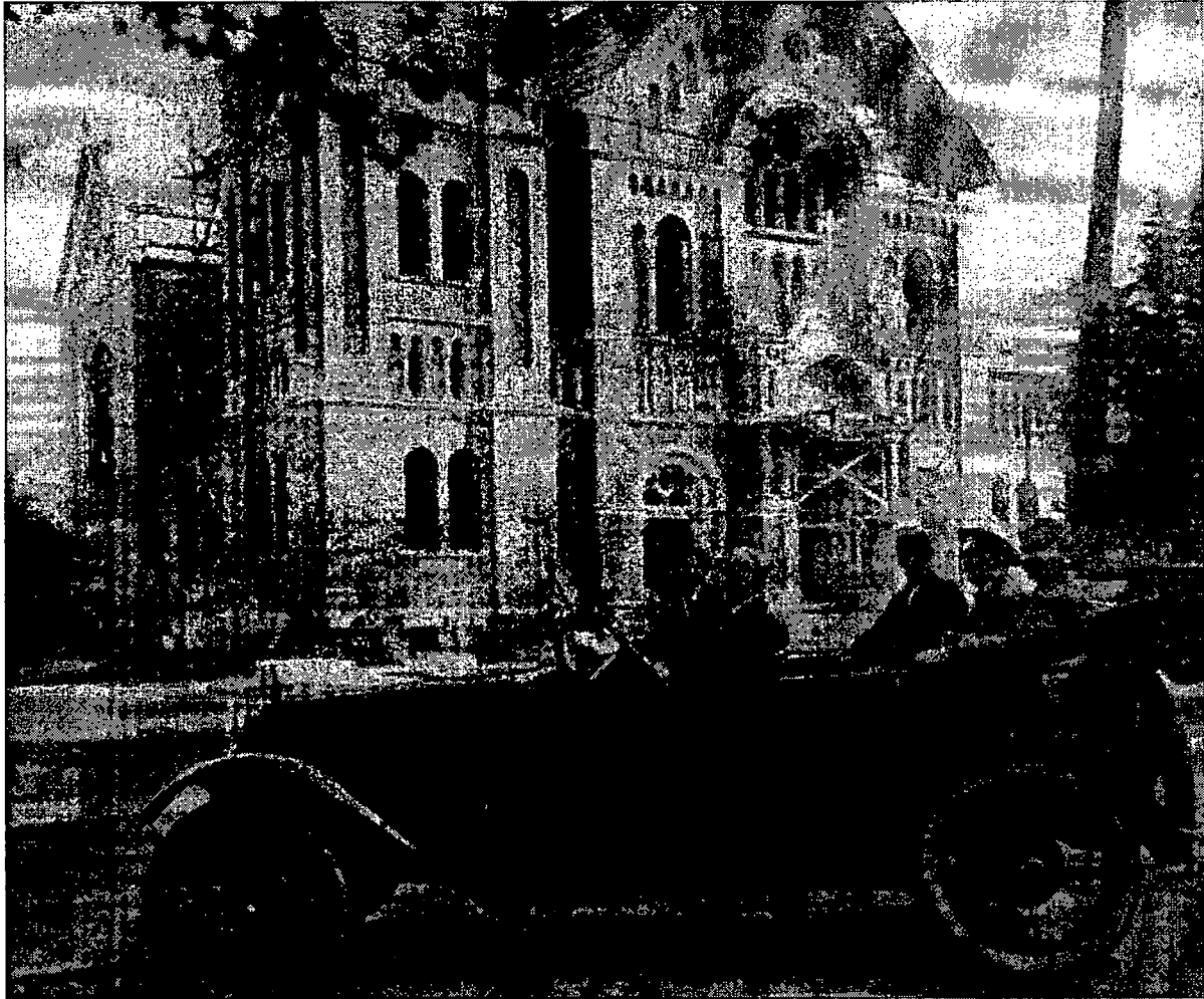
Historic photograph (dating from 1917) of the construction of St. Benedict Church on Irving Park Road. The gentleman in the rear seat closest to the photographer is Hermann J. Gaul, architect. Source unknown.
