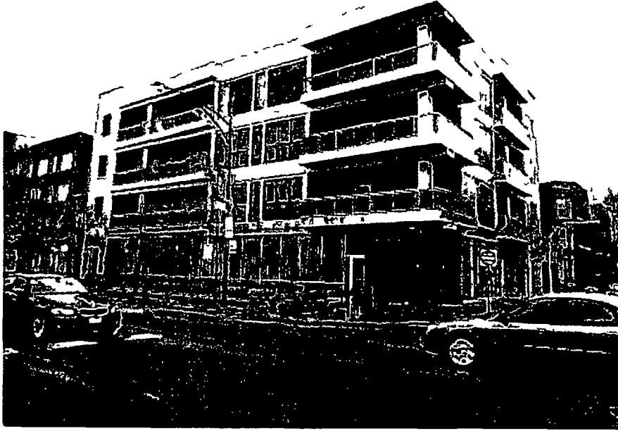
View of Southern Building Elevation
