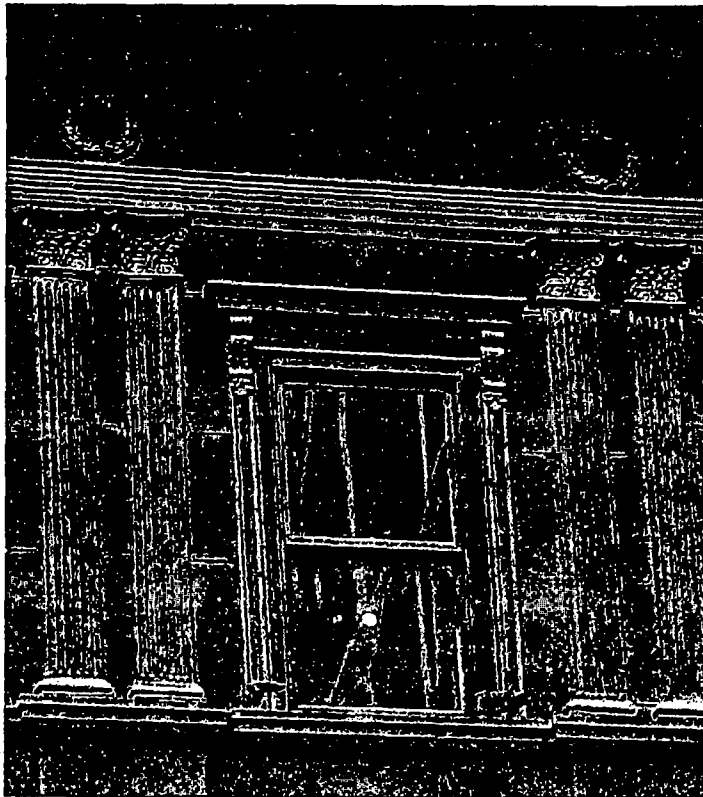
The west elevation of the west stationhouse (above) with the mezzanine level below it. The stationhouse exteriors are decorated with Neoclassical details (bottom left) rendered in pressed metal. Below right is one of the covered stairways which provide access to the Quincy Elevated Station.
