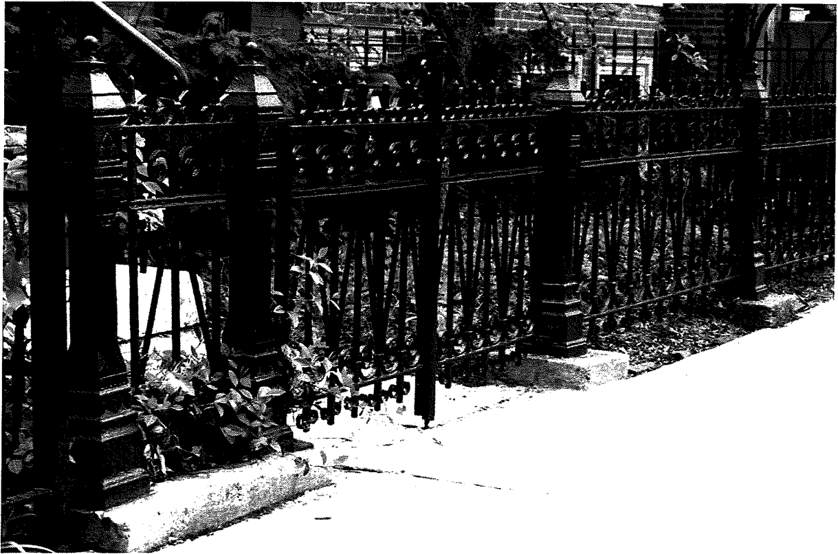
The Schnitzius Cottage retains all of its decorative-metal exterior detailing, highly unusual in the context of nineteenth-century Chicago residential buildings. Top: A view of the building's pressed-metal cornice, ornamented with brackets and dentils. Bottom: The building's cast- and wrought-iron front fence.
