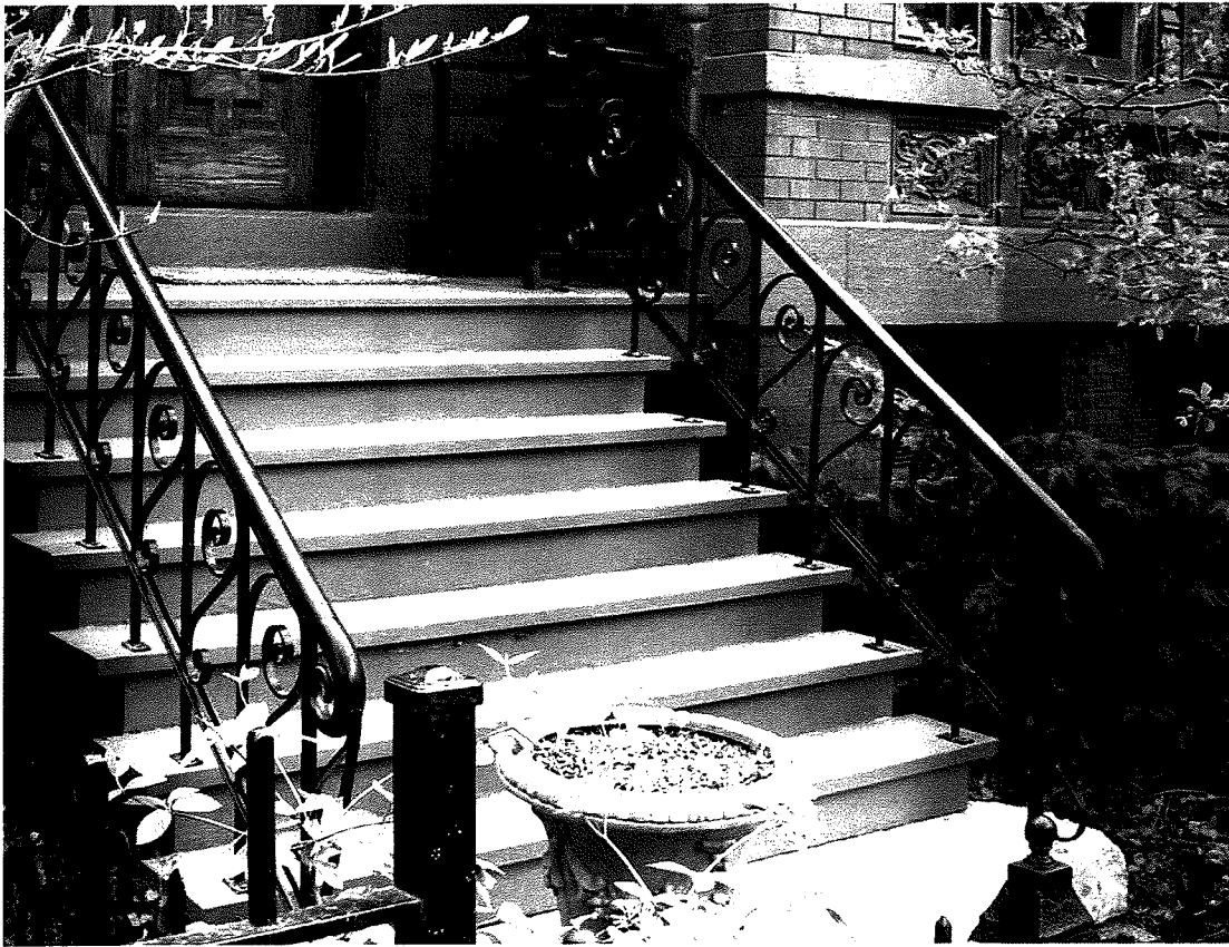
Details of the front porch's wood roof and cast- and wrought-iron railings.
