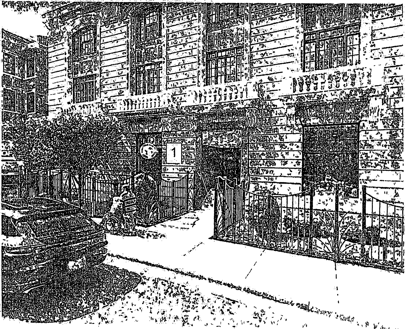
1 Belden looking northwest
