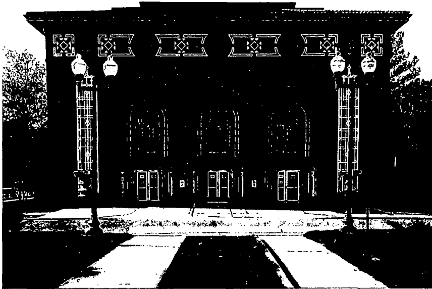
Main east elevation of the Auditorium Building.
