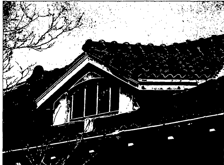
Above: Detail of the clay tile roof, dormer, and copper cladding. Left: Secondary entrance and stair tower on the east elevation. A cast stone urn (1917) is visible beside the doorway.
