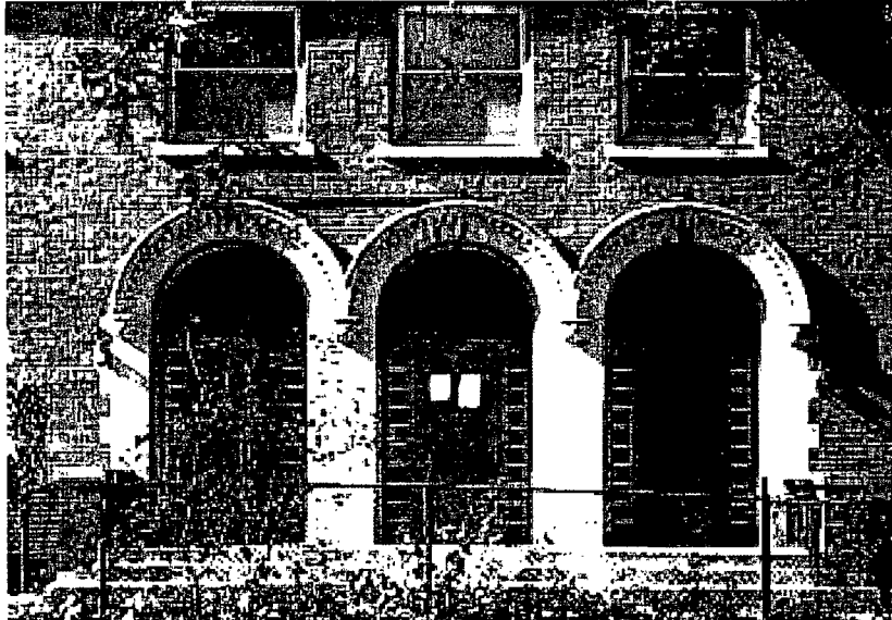
In 1924, a 2-story gymnasium wing was added at the southwest corner of the church building. Designed by architects Chatten and Hammond, the building is designed in a modest, twentieth-century variation on the Romanesque Revival style with a trio of round-arched entrances.
