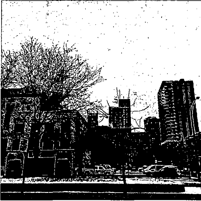
EXISTING PHOTO - LOOKING WEST
