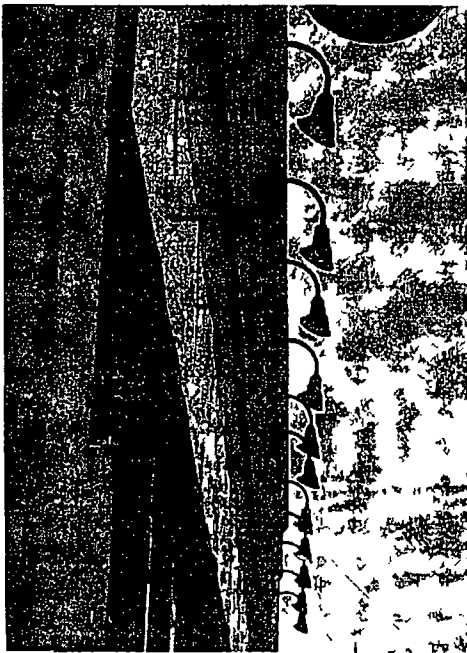
12 Goose neck 1 LAMPS on Lincoln Ave 183' length 183' width and 14.5' above grade
