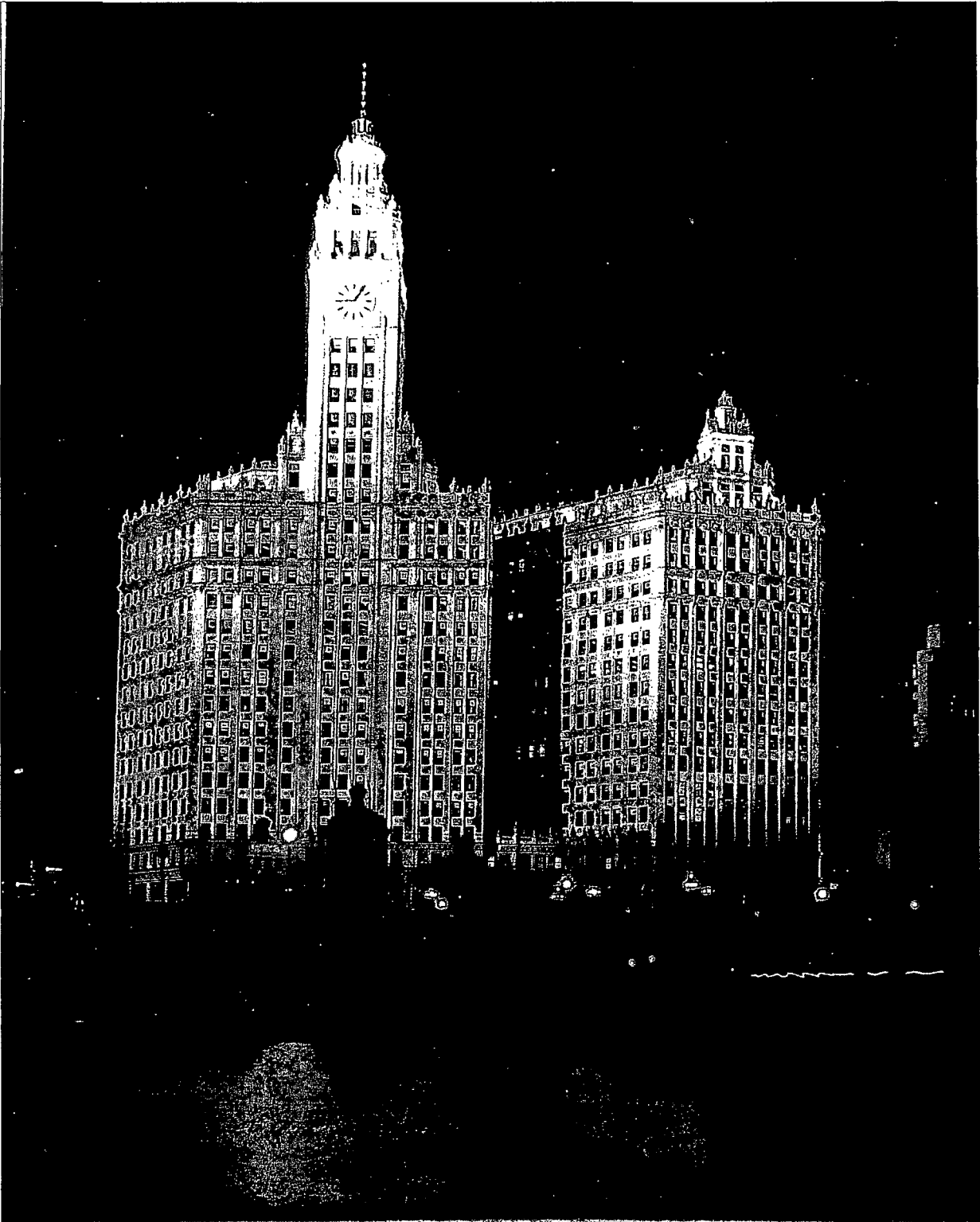
Night time illumination was a key component of the Wrigley Building's design, and it was one of the first skyscrapers to utilize an extensive lighting system. An innovative system of X-ray reflectors (later replaced by modern lighting) bathed the building in a brilliant light that made it visible for miles (Undated photograph from Wrigley archives).
