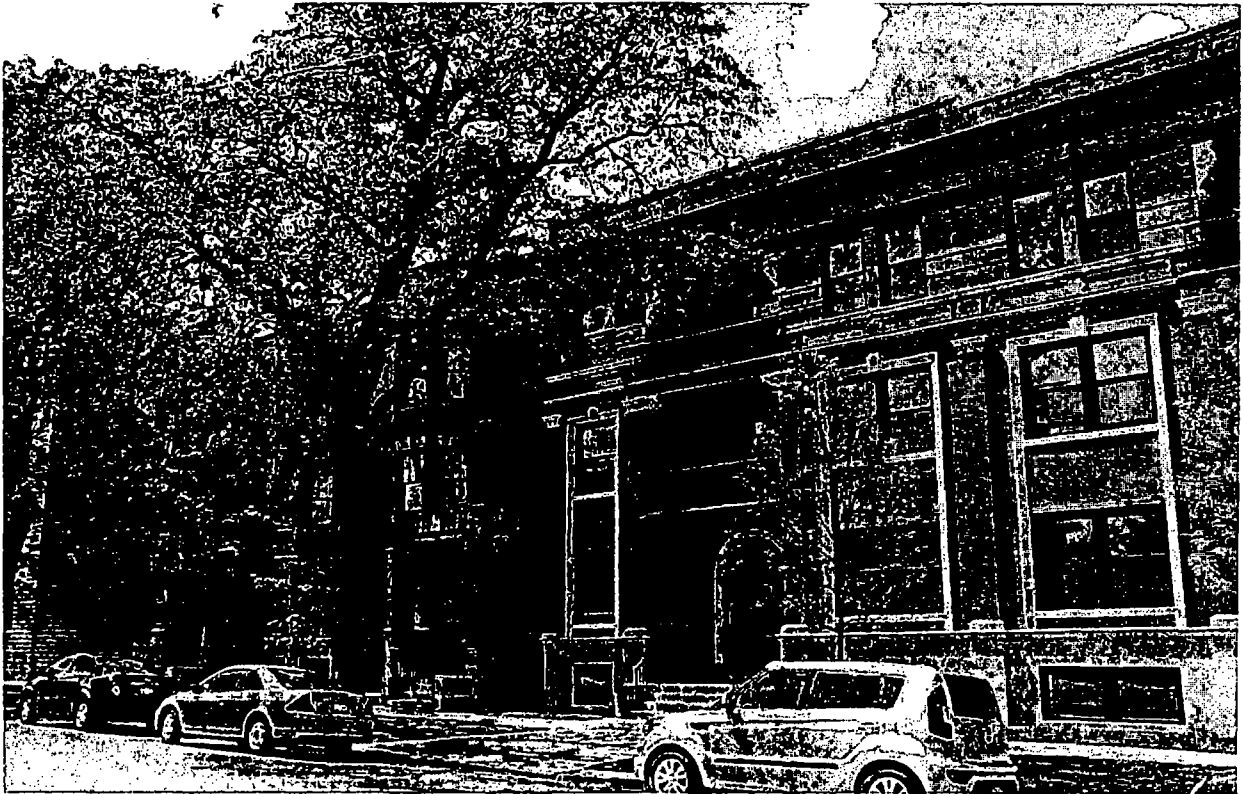
The Rosenwald Court Apartments are located on the block bound by S. Michigan Ave., Wabash Ave., S. 46th St., and S. 47th St. The 1929-30 portion of the building shown above, was commissioned by Julius Rosenwald. (Top) The garden apartment features a combination of Arts and Crafts brickwork with Art Moderne terra cotta detailing. (Bottom) The red brick apartment buildings were constructed in 1907 and 1908 and display elements of the Classical Revival style of architecture.
