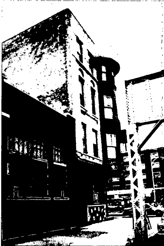
The north (Lake Street) and east (side) elevations of the (Former) Schlitz Brewery-Tied House located at 1393-1399 West Lake Street, 1987. The faded paint of a sign including the trademark Schlitz font logo can be seen on the east elevation. (Survey card, Chicago Historic Resource Survey )
