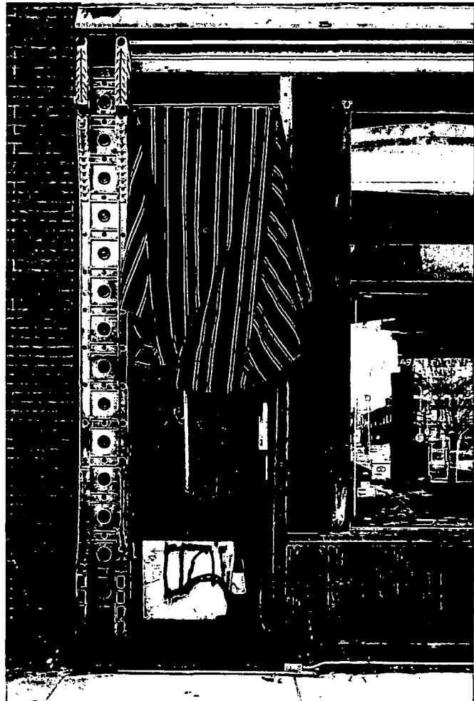
Cast iron structural members frame the original storefront opening including a decorative pier, lintel, landings, and sills. Photo of the north elevation. (Photo by Patrick L. Pyszka)
