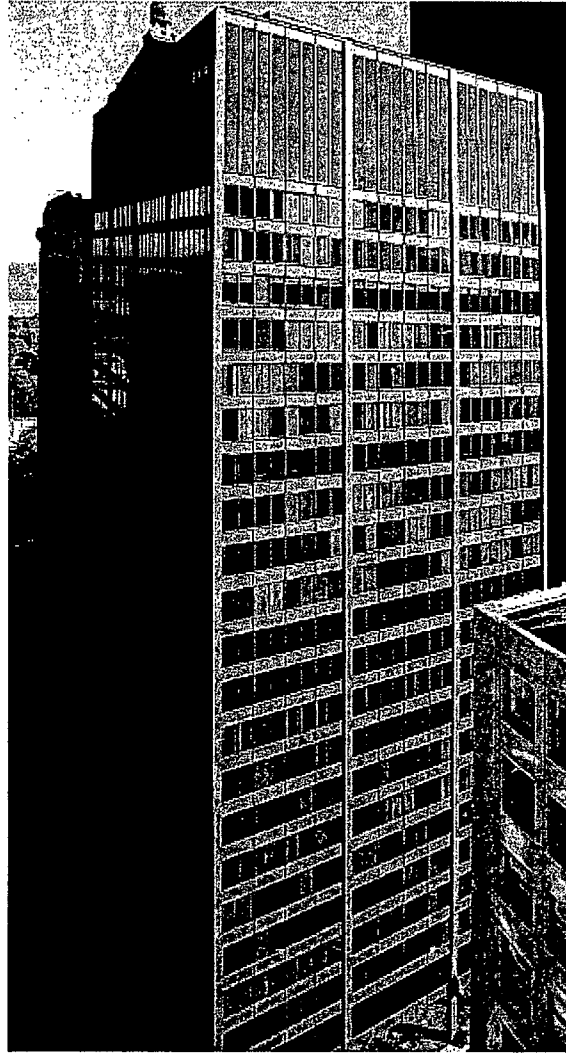
The Continental Center remains an outstanding example of a glass-and-steel skyscraper designed in the International Style and has excellent exterior integrity. The steel curtain walls and original gray-tinted windows remain intact, as do the glass walls enclosing the lobby and the steel structural columns at the building's base.
