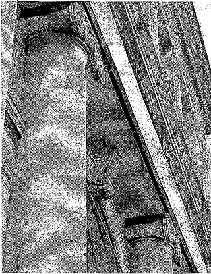
Details of the Ionic column capitals and soffit of the temple-front entrance portico (left) and of the entablature on the east elevation (below) illustrate the building's fine detailing and craftsmanship in carved limestone.
