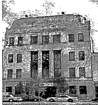
CHICAGO CITY BANK AND TRUST 815 W. 63rd Street Date: 1930 Architect: Abraham Epstein
