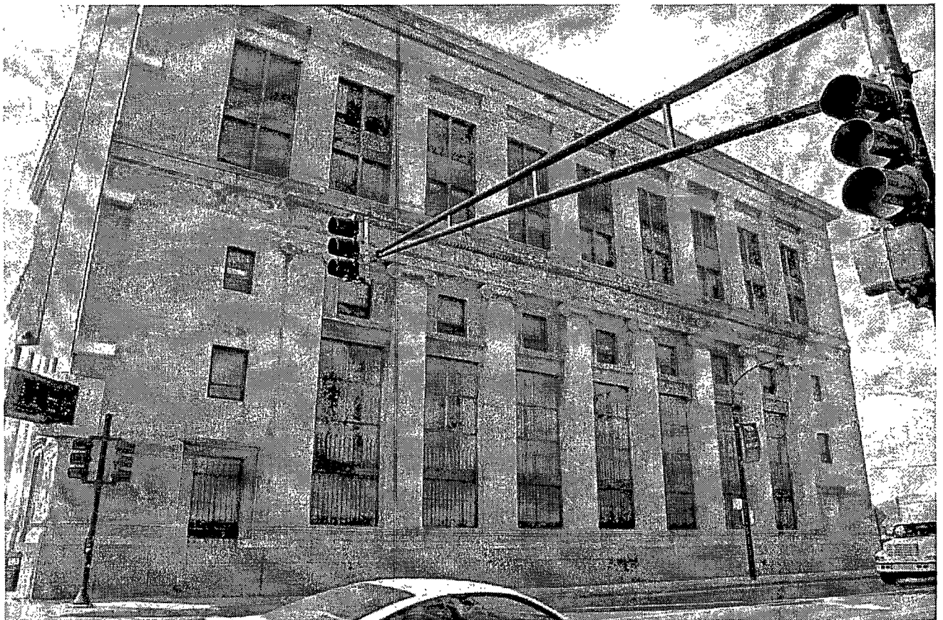
The side elevation facing Pulaski Avenue (bottom) reflects the internal function of the building. The triple height banking hall is illuminated by the large windows at the base of the building. The smaller windows at the upper stories were designed for commercial offices on floors four and five.
