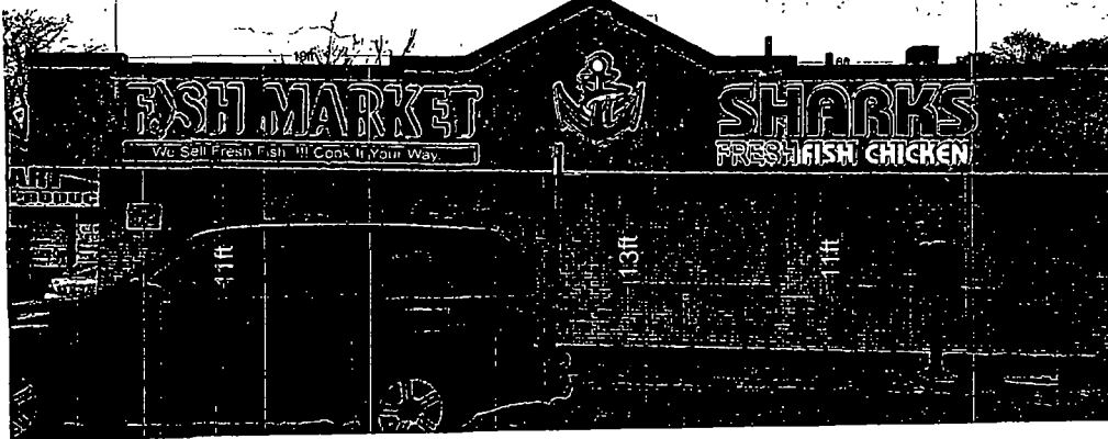
Front Sign face to 71st Street
