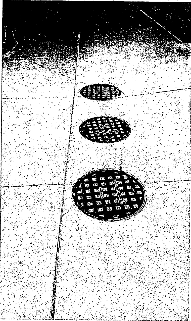
Grease Trap located on Milwaukee and Clinton (center)
