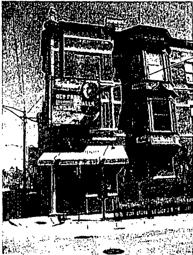
Looking north at south face of building
