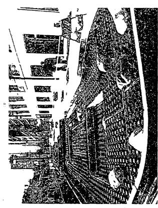
Existing Planter Construction. The existing 7 planters vary in size and provide approx. 1.800 cubic feet of soil for 10 trees, equivalent to 180 cubic feet per tree. Although the planters have a large footprint, they only have +1-12 of soil depth throughout, with the remainder filled with insulation. Tree pits are carved out of the insulation to provide +1-12 of additional soil for the trees.
