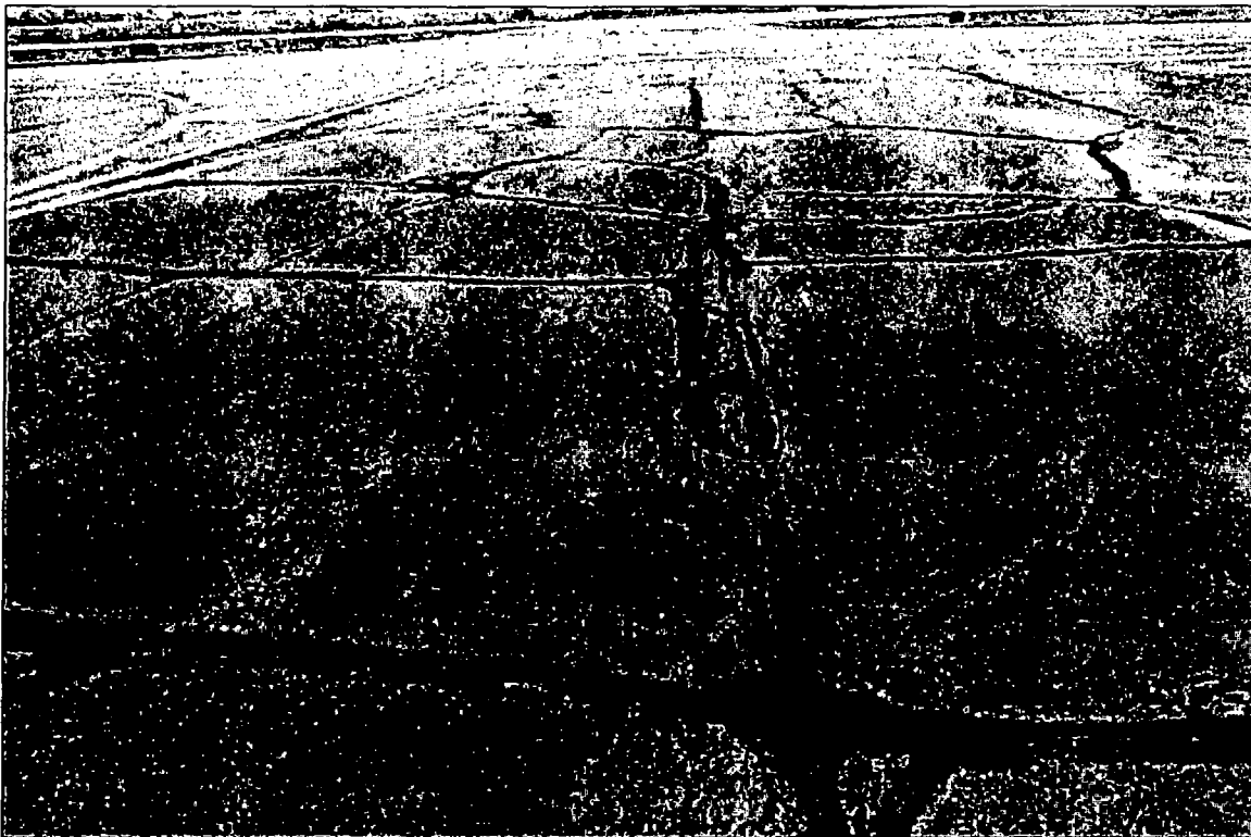
Figure 2-6. Typical Poor AC Pavement (Feature 170)
