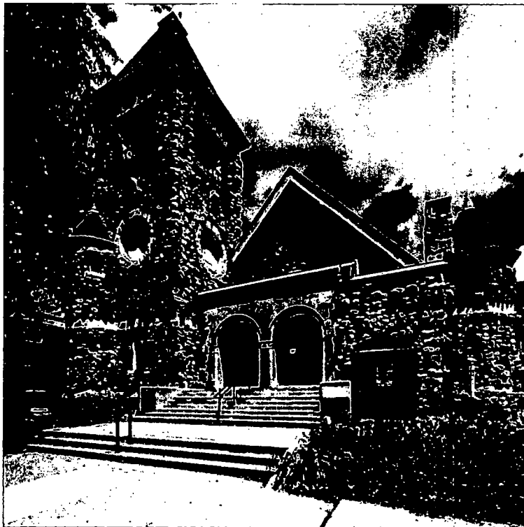
The facade of the church showing the distinctive uncoursed fieldstone walls built of natural granite boulders. The gable front is framed by projecting, asymmetrical towers. The arched entrance doors open up into an enclosed vestibule, or narthex, added in a 1930 renovation.
