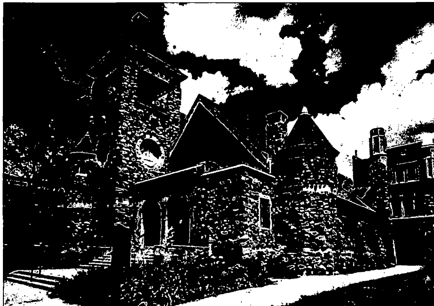
Epworth 2022, showing the addition of the narthex and a partial view of the community house addition which are historically significant changes.
