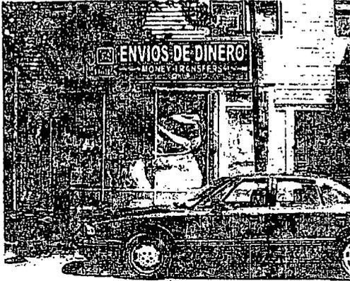
SIGN IS MOUNTED 120" ABOVE GRADE TO THE BOTTOM OF SIGN
