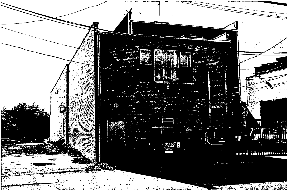
4321 S. Cottage Grove Avenue – Rear South Side
