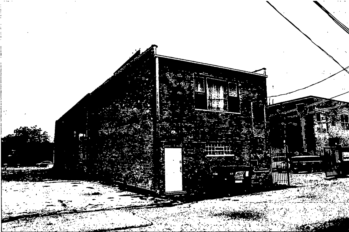
4321 S. Cottage Grove Avenue – Rear South Side
