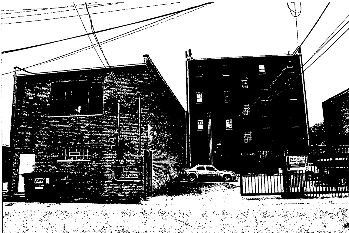
4321 S. Cottage Grove Avenue – Rear North Side
