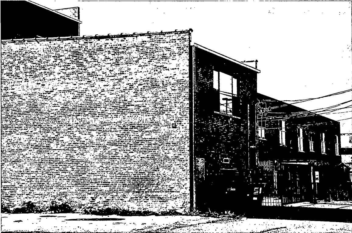
4321 S. Cottage Grove Avenue – Rear South Side
