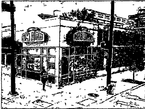
TWO IDENTICAL SIGNS SHOWN ON BUILDING
