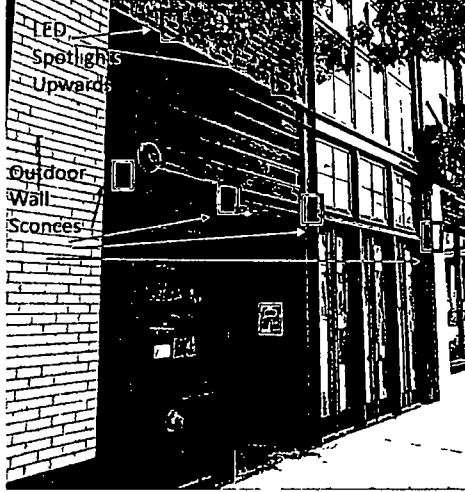
733 N LaSalle – Front Entrance View
