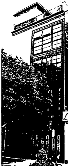
733 N LaSalle – Building Face
