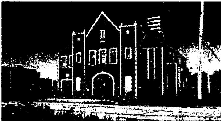
Package B1/B2 - Firehouse Site (Existing)
