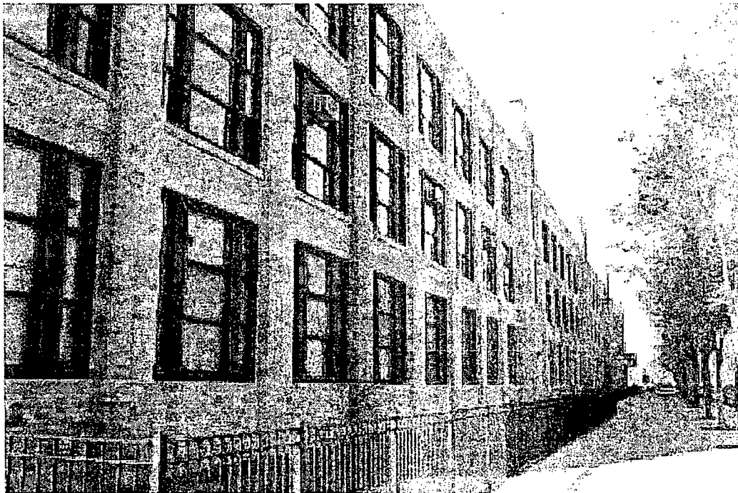
Above: Limestone banding outlines rows of windows and delineates piers on the State St. elevation.
