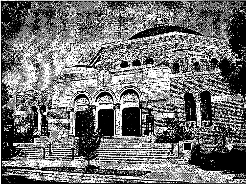
Site Photograph of 5039 S. Greenwood Avenue Temple Entrance Source: Open House Chicago 2015, Eric Allix Rogers, Photographer
