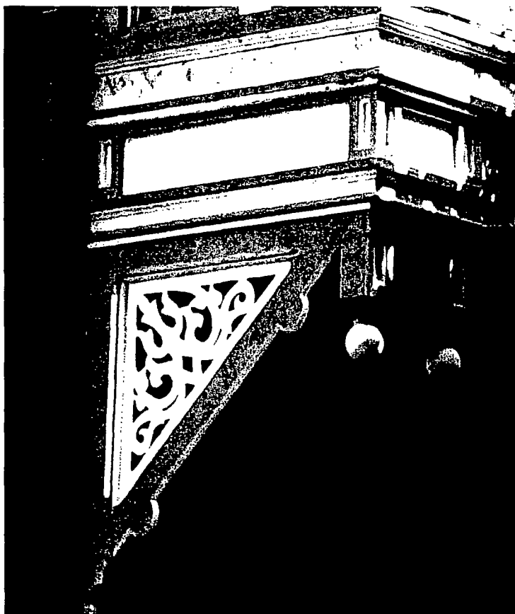
The Warner House also has an unusual second-story projecting bay paneled and decorated in wood. Left: The bay is supported by pairs of carved-wood brackets detailed with curvilinear "jig-saw" ornament. Top: The bay is also ornamented with wood panels and a bargeboard detailed with scalloped edging.
