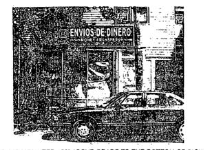
SIGN IS MOUNTED 120" ABOVE GRADE TO THE BOTTOM OF SIGN AND EXTENDS 10" OVER PUBLIC WAY 10"-2" FROM OUTER EDGE OF SIGN TO CURB LINE
