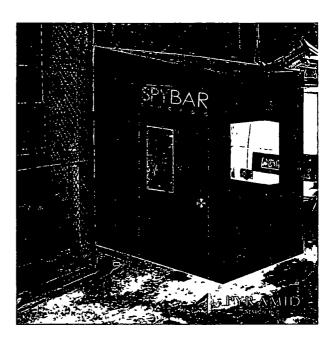
Existing Windscreen to protect staff and patrons from weather. (101" Height x 10' length along the public way 7' over public way) 1 Windscreen constructed of 1" galvanized steel square tube. 2 doors, clear vinyl windows.
