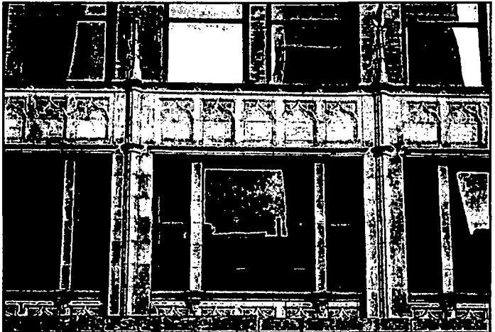
The Dearborn Street elevation of the Plymouth Building, remodeled in 1945 for the LaSalle Extension University, combines original brick-and-terra-cotta detailing by Eisendrath with later Collegiate Gothic-style architectural terra cotta manufactured by the Northwestern Terra Cotta Company, which was founded in Chicago in 1878 and became one of the leading terra-cotta manufacturers in the country. The company supplied architectural terra cotta for important Chicago buildings including the Civic Opera House and the Chicago Theater.
