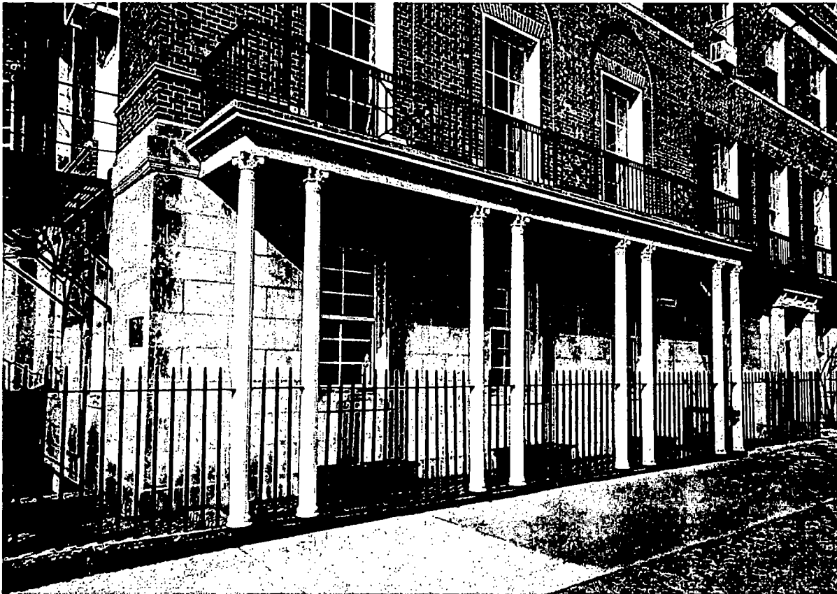
Image 40: Detail of cast-iron columns and balcony of number 2700.
