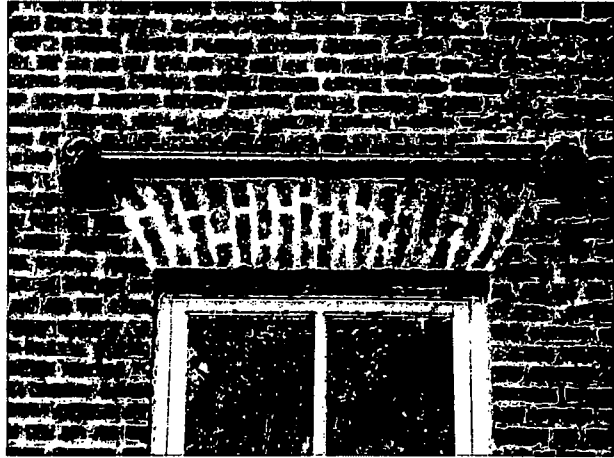
The later corner tower addition has flat arches with decorative red terra cotta drip moulds and foliate label ends. One larger terra cotta producer was the Northwestern Terra Cotta Company, which was founded in Chicago in 1878.
