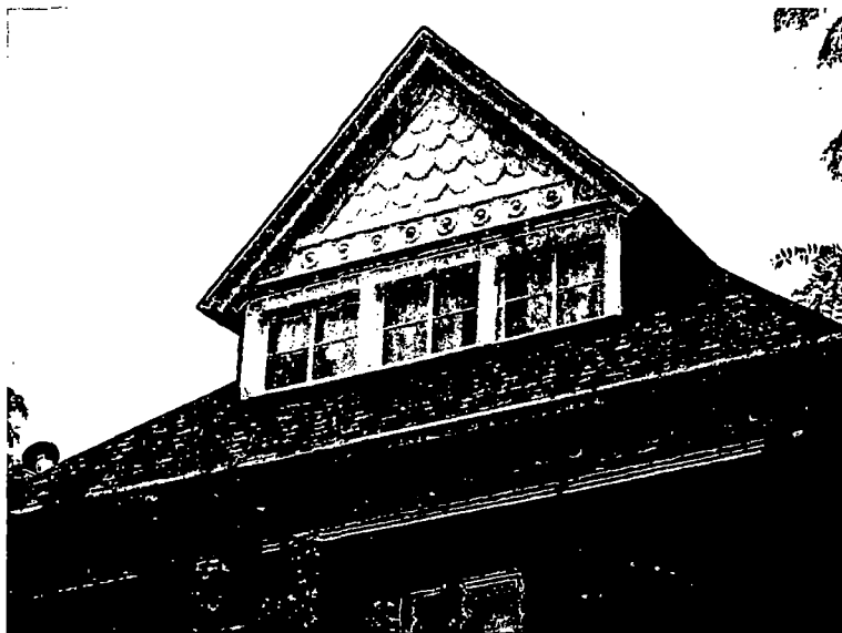
The south addition features a west-facing dormer and pressed metal cornice and pediment with Queen Anne style details.
