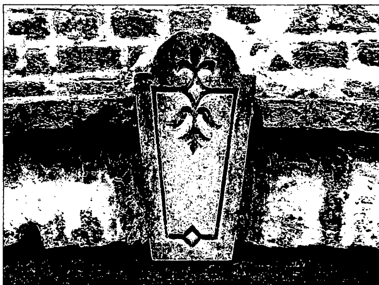
The gables of the original portions of the house feature cast stone keystones with deeply incised details.
