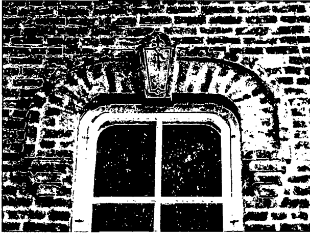
The original portion of the house features brick window hoods with cast stone keystones. Cast stone is a cementitious artificial stone that was widely produced in Chicago after it was patented by George A. Frear in 1868.
