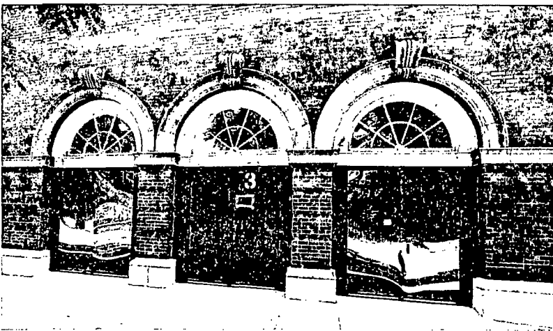
The 1923 addition has fine examples of Classically-inspired ornament. At left is shown a trio of entrances on the west elevation that lead to auditorium. Each is bordered in unglazed terra cotta and features a prominent keystone in the shape of a scroll.
