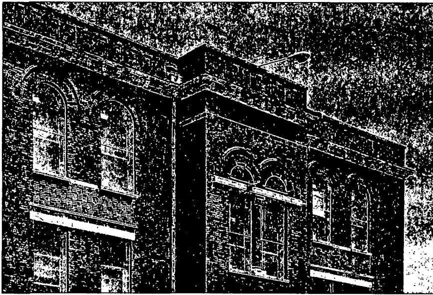
Left: The south elevation of Fiedler's 1894 building features decorative molded brick and fine arched terra cotta hood molds with foliate returns. The central bay features a twin stairwell window with a brick column as a mullion.
