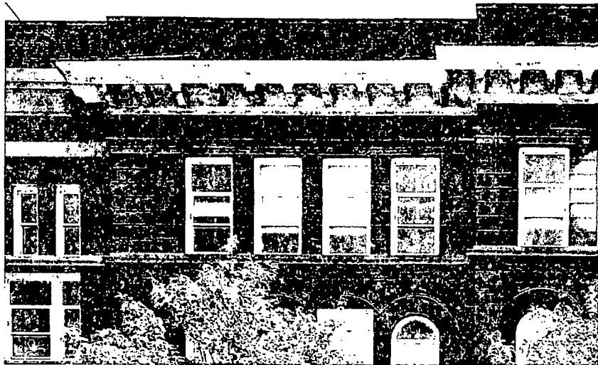
Right: The 1900 addition is similar to the 1894 section, but it includes a third floor with Classically-inspired details. Rusticated brickwork and a large metal cornice top the addition.
