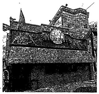
Custom Flat Mounted Sign Mounted with 8 3/8" Lag anchors to brick wall 2 5" bolts through L brackets mounted to sign
