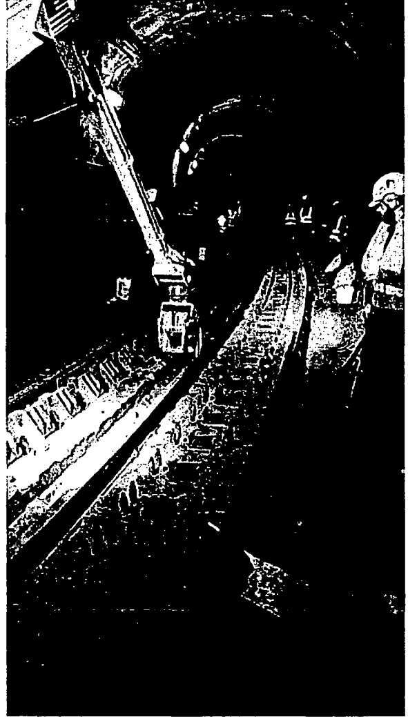
Replacing plates and 80 pieces of rail at Clark/Division
