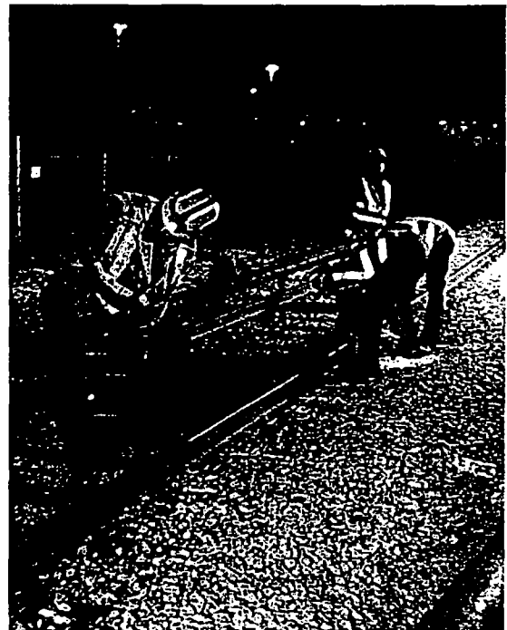
Spiking gage ties and securing track with screw spikes Blue Congress Branch
