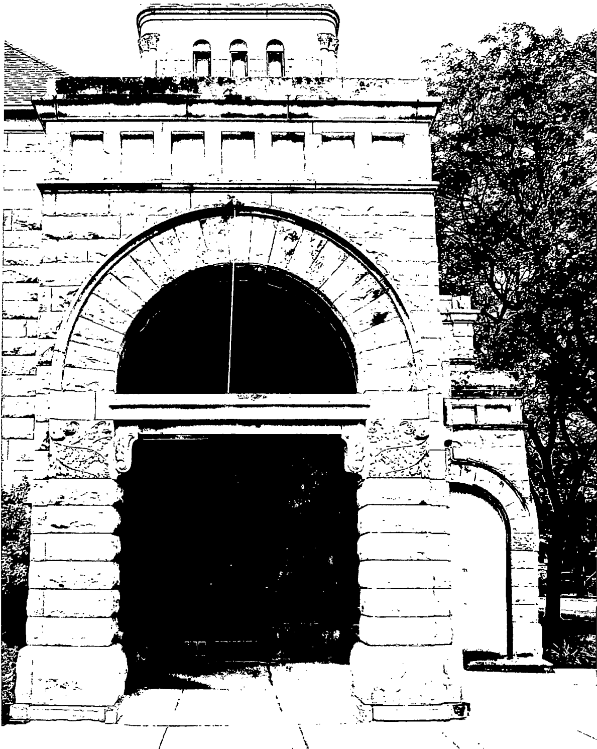
The double-arched portico to the east of the main entrance bay features round-arched openings and a paneled cornice. Profiled limestone lintels supported by acanthus-ornamented brackets span the bottom of the arches.
