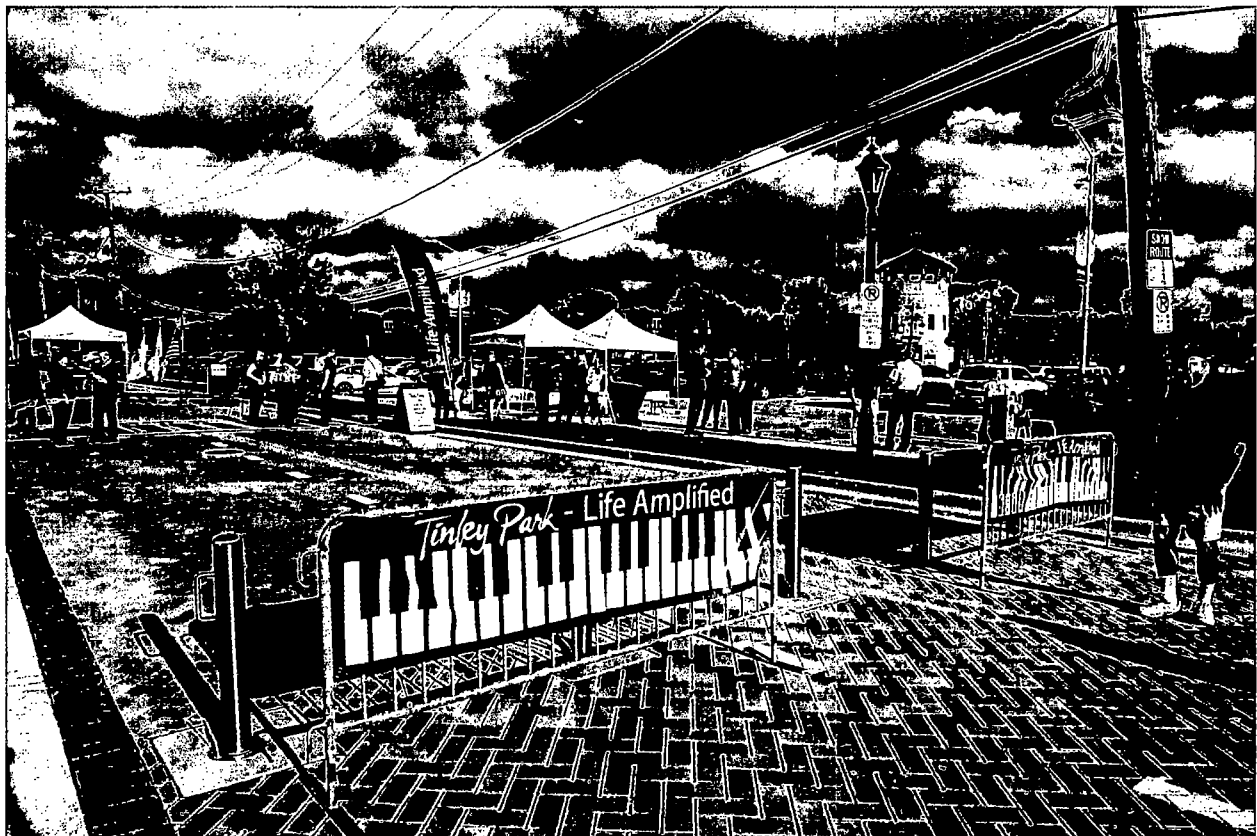
A new permeable paver project on North Street in Tinley Park was unveiled by MWRD Commissioners Debra Shore and Kim Du Buclet along with Tinley Park officials in October as part of the Harmony Square development near the Metra Station. The MWRD contributed $200,000 to replace asphalt with 16,500 square feet of permeable pavers on North Street, which will provide more than 69,000 gallons of stormwater storage on site.
